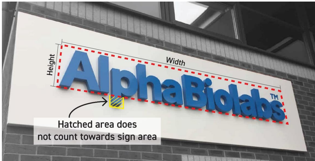
Figure 22: Example Illustration of letter descenders that are not counted toward the sign area
